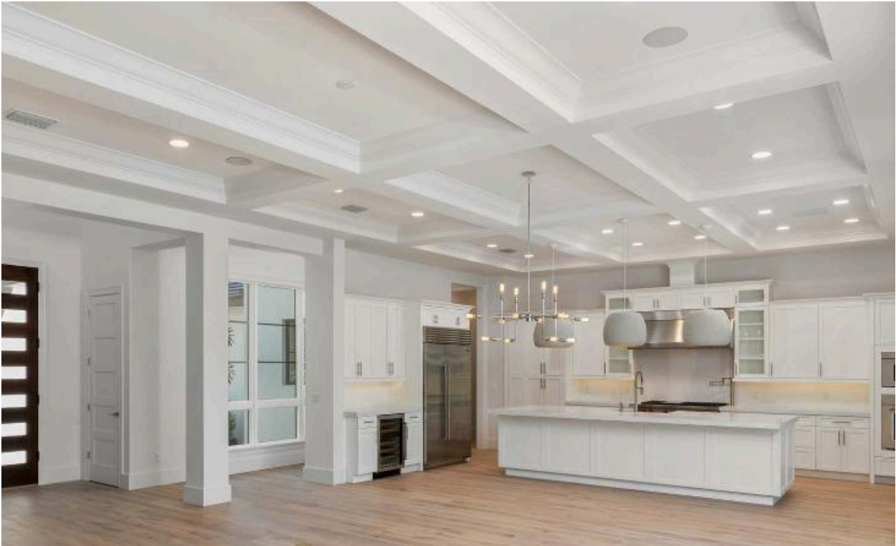
Drywall Coffered Ceiling with Added Crown
