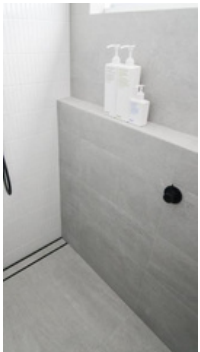
Shower Ledge Left Side Shower Wall Approx 48"H
