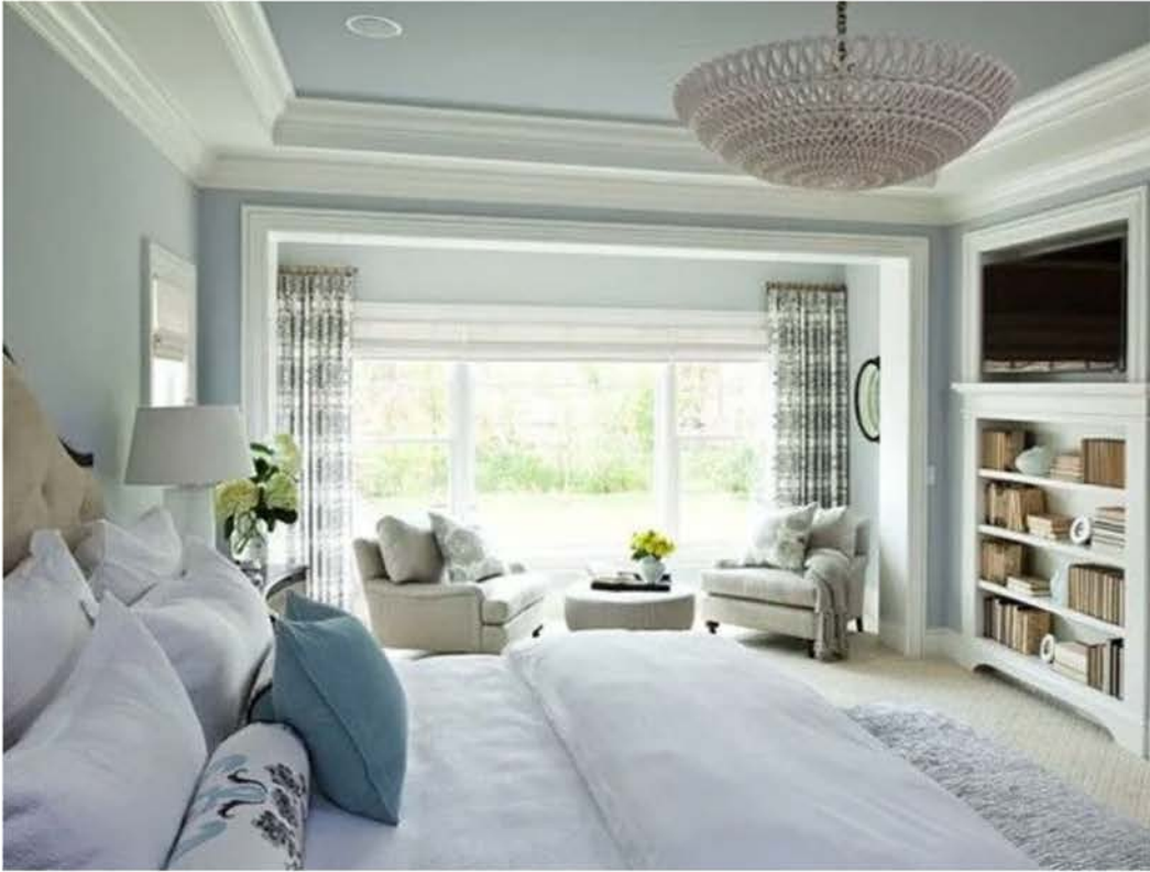
CONCEPT PHOTO Tray Ceiling & Crown Inside & Outside of Tray
