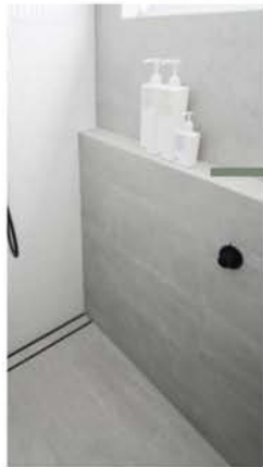
SHOWER LEDGE Same Shower Wall Material *Run Length of Back Wall, Approx 48" H
