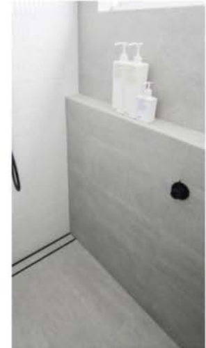
SHOWER LEDGE Same Shower Wall Material *Run Length of Back Wall Approx 48" H
