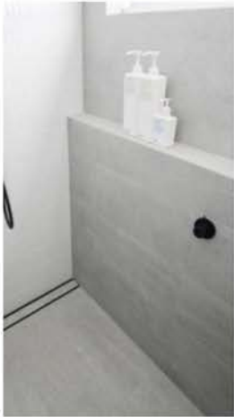
SHOWER LEDGE Same Shower Wall Material *Run Length of Right Side Facing Wall Approx 48" H
