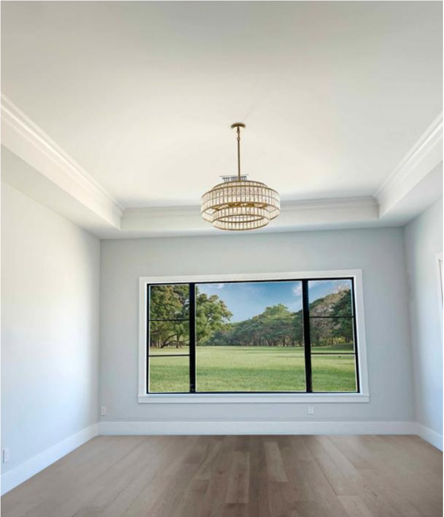
Soffit/Tray Ceiling W/ Added Crown
