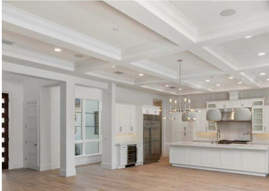
DRYWALL COFFERED CEILING Painted W/ Added Crown
