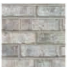
FRONT PORCH BRICK FLOORING Knob Hill
